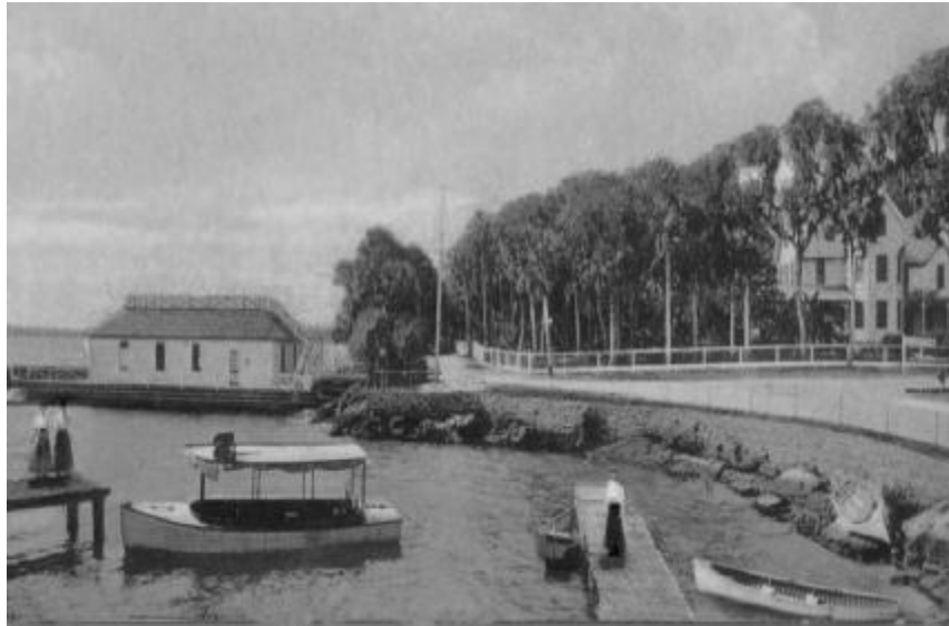
In the picture above, ladies stroll on the docks along the Indian River near the big hotels of Rockledge. The W. H. Rankin residence still stands at the corner of Rockledge Drive and Barton Avenue.
