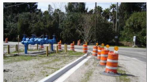
Gas Meters at John Rodes Blvd.
