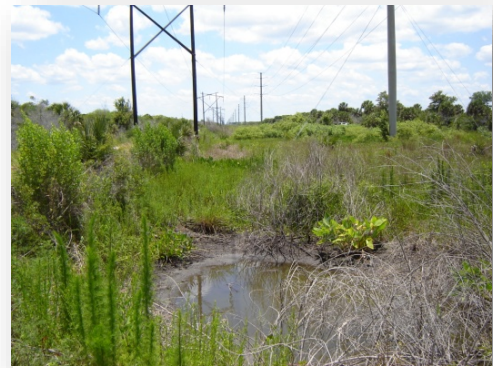
Existing Utilities Along I-95
