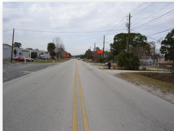
Existing Ellis Road
