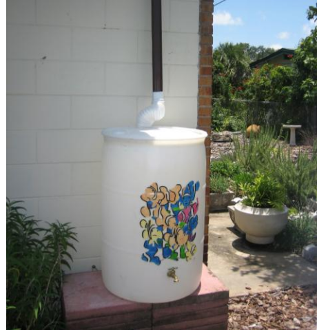
Colorful Rain barrel in collecting downspout run-off Photo by: Diane Dougherty, Homeowner
