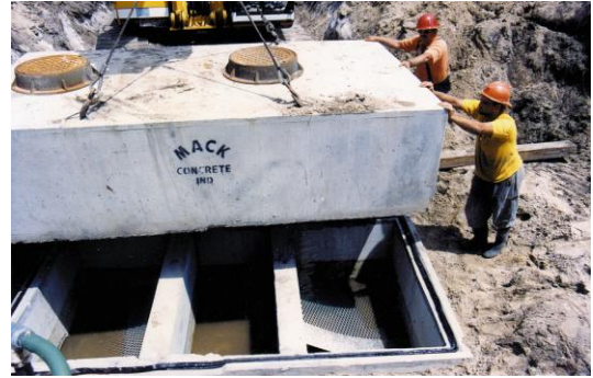
Installing a Baffle Box to reduce sediment and nutrients entering the Lagoon Photo by: Greg Jones, Brevard County NRMO
