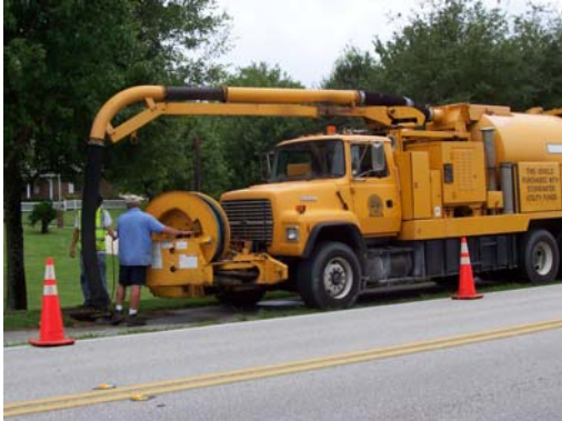
Cleaning out sediment and debris from the storm drain Photo by: Greg Jones, Brevard County NRMCO
