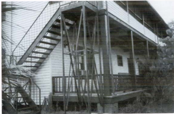
TAMARIND, PRESENT DAY SHOWN WITH ITS STEEL FIRE ESCAPE
