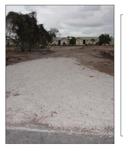
A stone stabilized pad located at points of vehicular ingress and egress on constructio n sites reduce the amount of sediment transported to public roads by motor vehicles or runoff.
