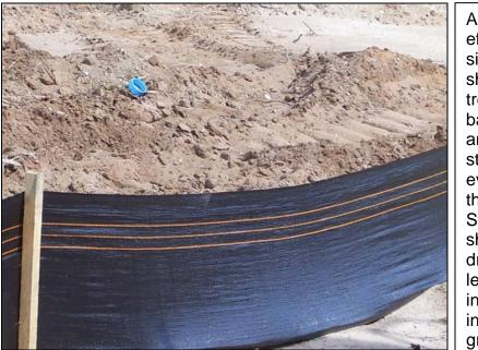
An effective silt fence should be trenched, back filed and staked every three feet. Stakes should be driven at least eight inches into the ground.
