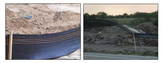
Examples of BMPs: Silt fence on the left is a properly maintained silt fence. On the right is an improperly maintained silt fence. It does not prevent sediment from leaving the construction site. Below, storm drain on the left allows pollutants to enter. A prefabricated drop inlet external filter stops pollutants from entering the drain.
