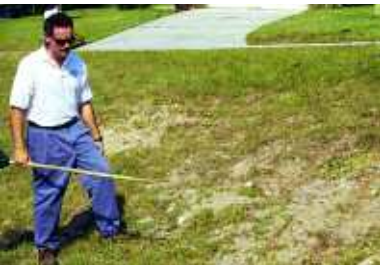
Repair eroded slopes.
