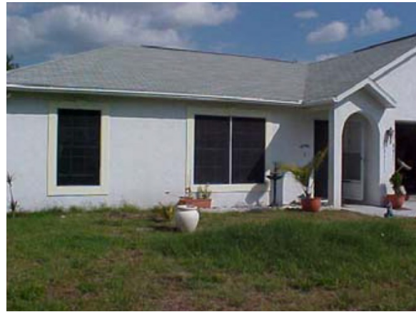
Figure 4 - After. House with solar screens.
