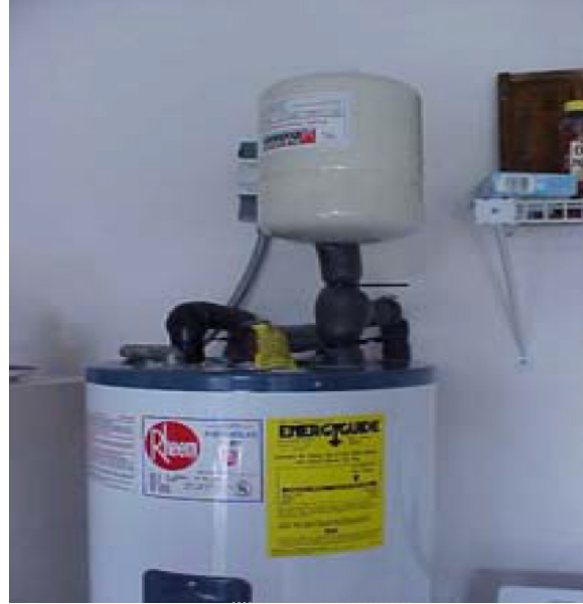
Figure 6 - After. New, gas water heater.
