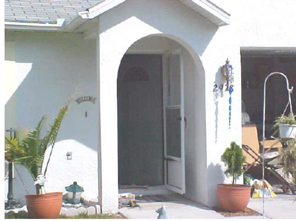
Figure 2 - After. New front door and screen door.
