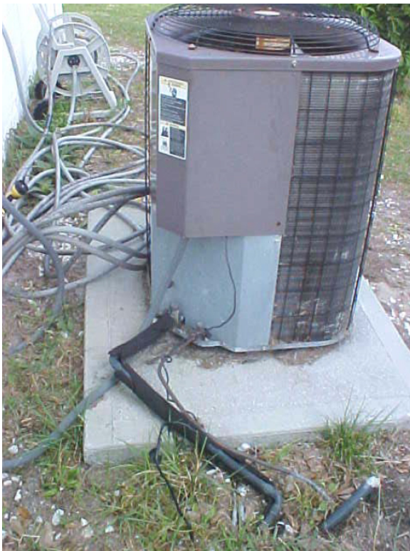
Figure 7 - Before. Outdoor air conditioning unit with exposed, worn out pipes.
