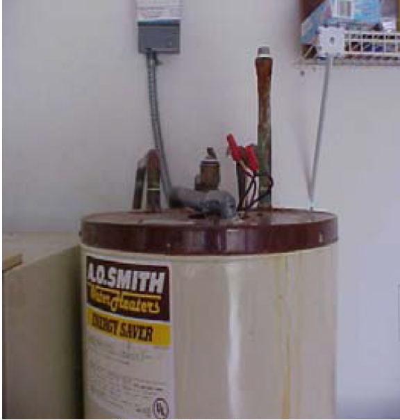
Figure 5 - Before. Old, rusted, electric water heater.
