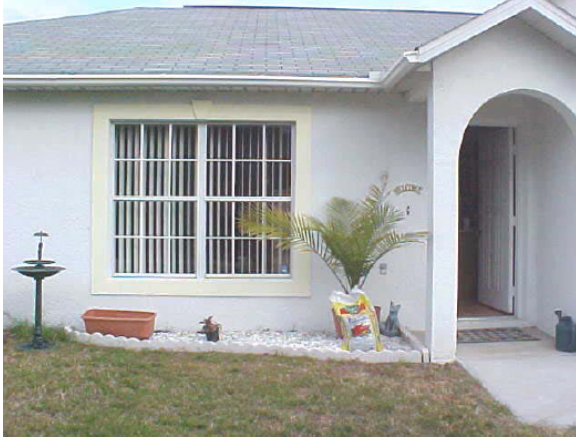
Figure 1 – Before. Old front door.
