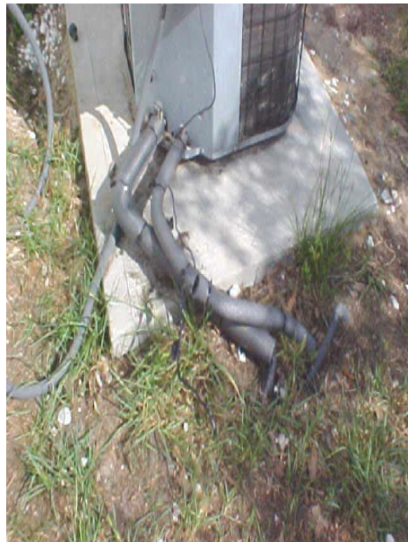
Figure 8 - After. Outdoor air conditioning unit with weatherized pipes.
