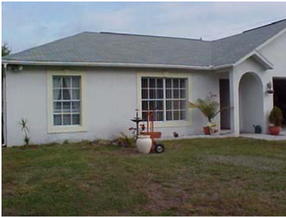
Figure 3 - Before. House without solar screens.
